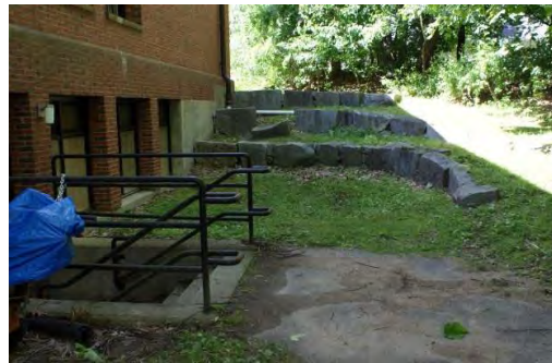
Rocky slope to the Stairwell
