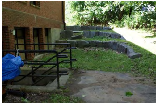
Rocky slope to the Stairwell
