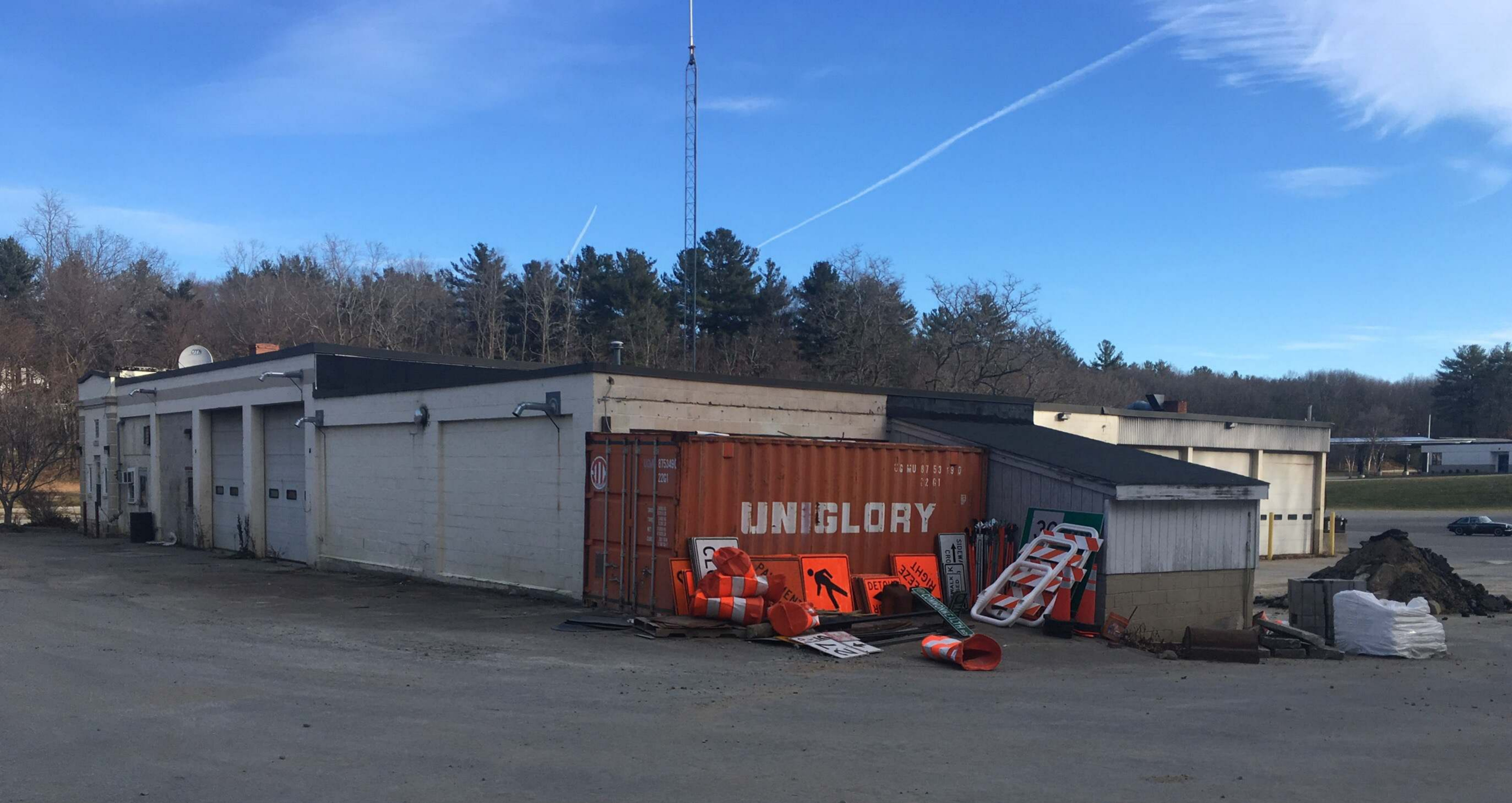
View of main structure from the southwest
