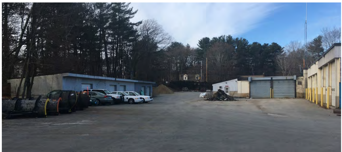
View of both existing buildings looking west.
