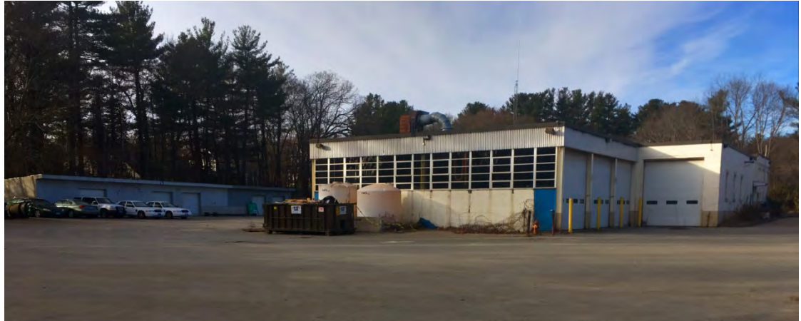
View of existing structures, garage, and shed, from the south.
