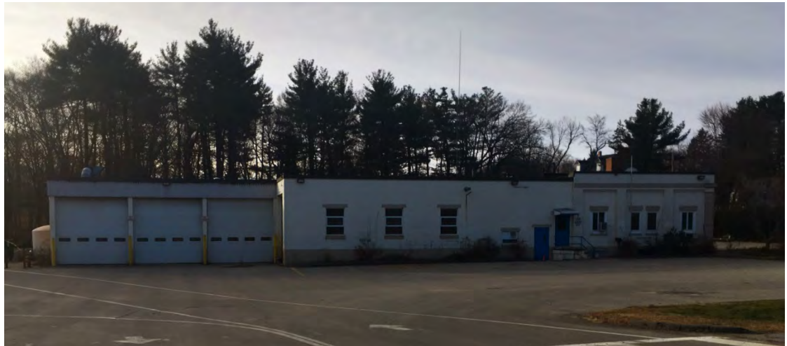
View of existing highway garage from the driveway.
